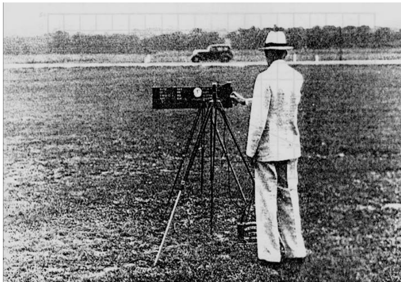
Fig. 2: Greenshields measurement set up for the reported 75 years ago
